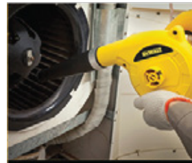
The textile mill blows dust
